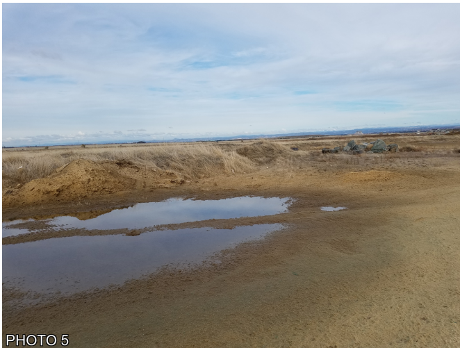
PHOTO 5 SOIL AND ROCK STOCKPILES IN VILLAGE 3B
