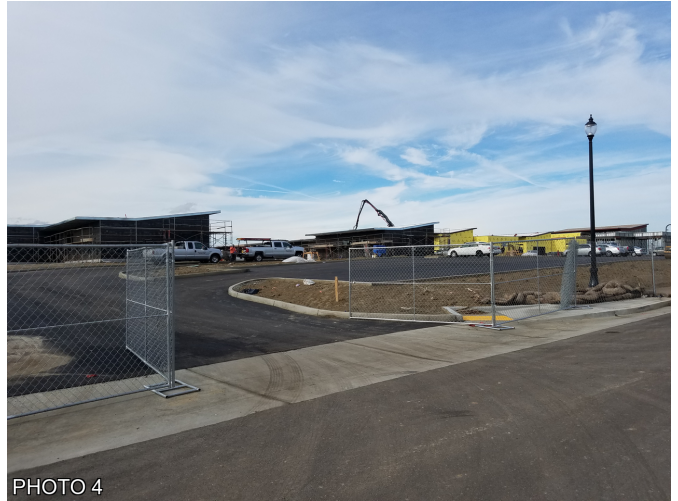
PHOTO 4 RIEGO CREEK SCHOOL CONSTRUCTION IN EAST PORTION OF VILLAGE 3A
